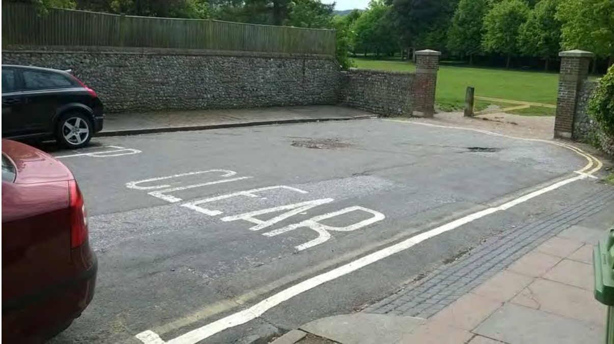
View 3 – Looking westwards across Saffrons Road
