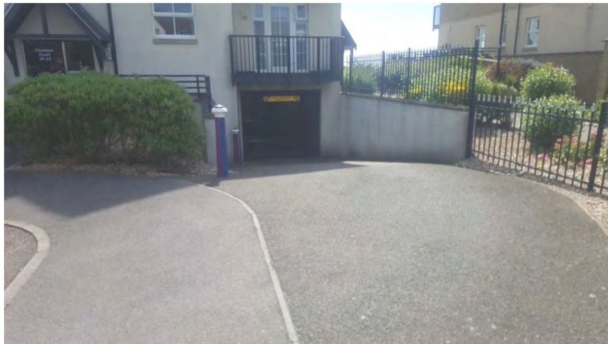
View 7 - Looking south-eastwards towards underground car park entrance
